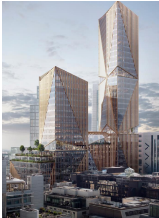
2 Finsbury Avenue, London
